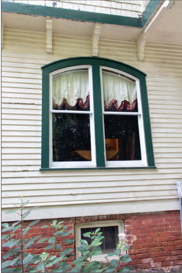
Figure 3.5. First-Story, Segmental-Arch Window, Facing South
