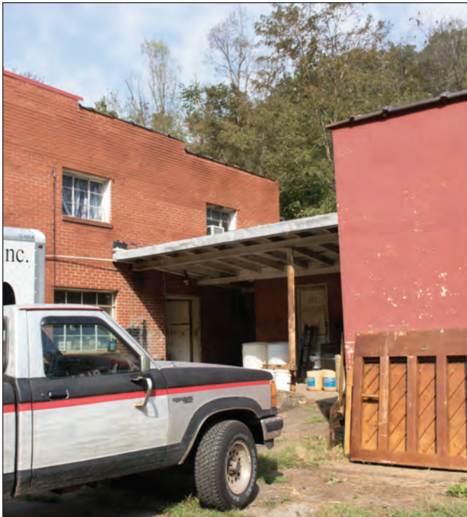
Figure 6.6. Breezeway Between Factory and Workshop, Looking Southeast
