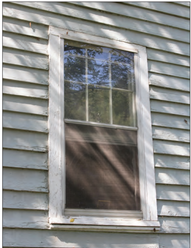
Figure 5.11. Sash Window, Facing West
