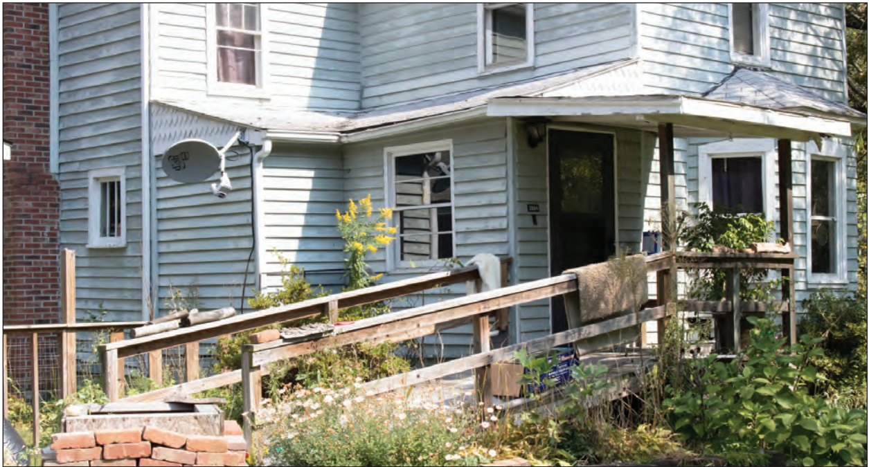
Figure 5.12. Entrance and Enclosed Porch, Facing Northeast
