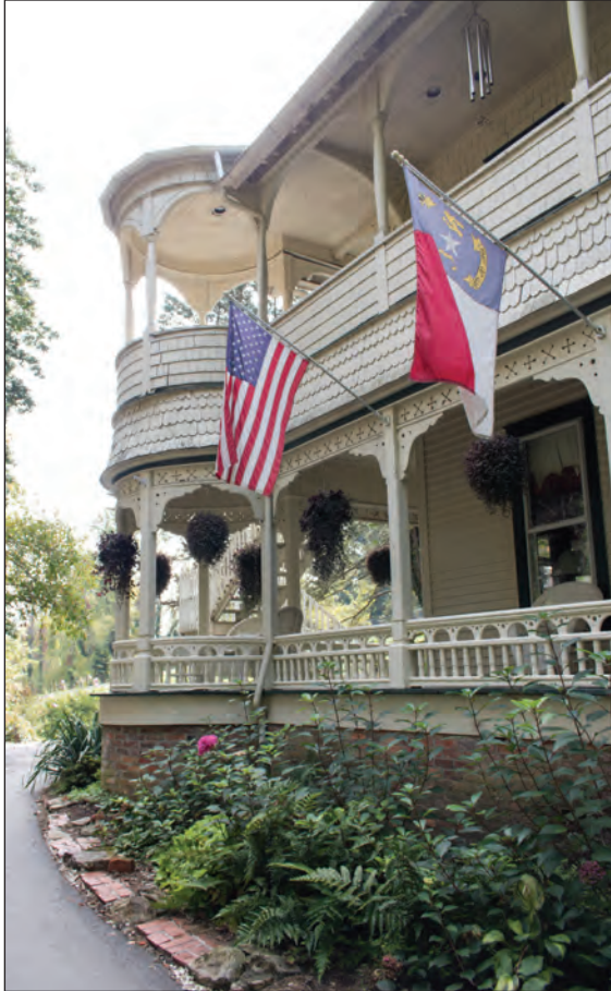
Figure 3.3. Turret and Porches, Facing East
