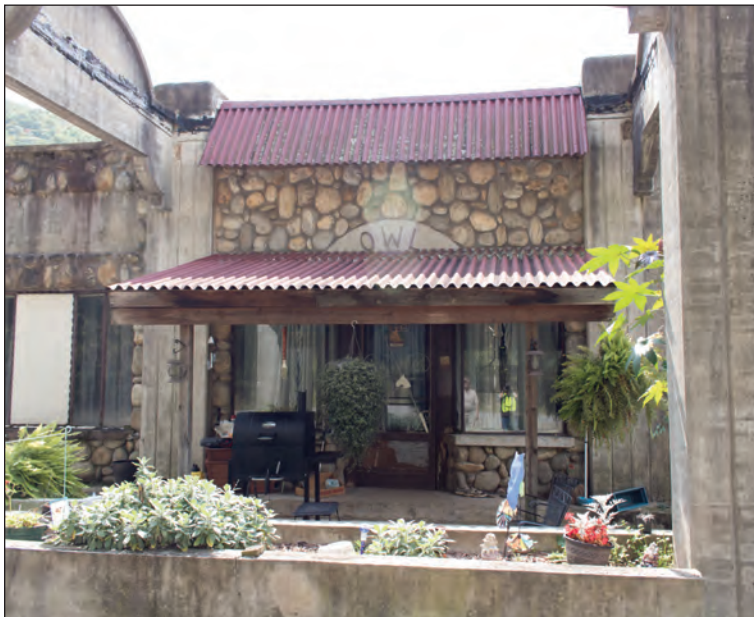
Figure 4.6. Center Bay of the Façade, Looking South
