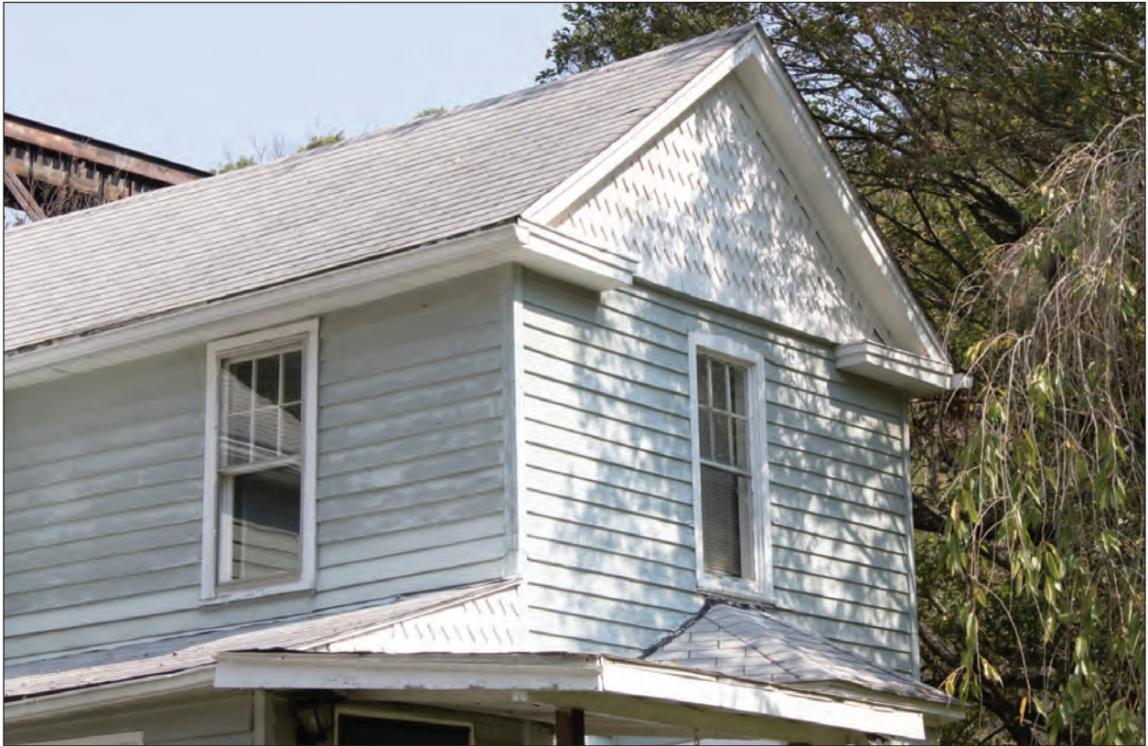
Figure 5.9. Patterned Shingles, Facing Northeast
