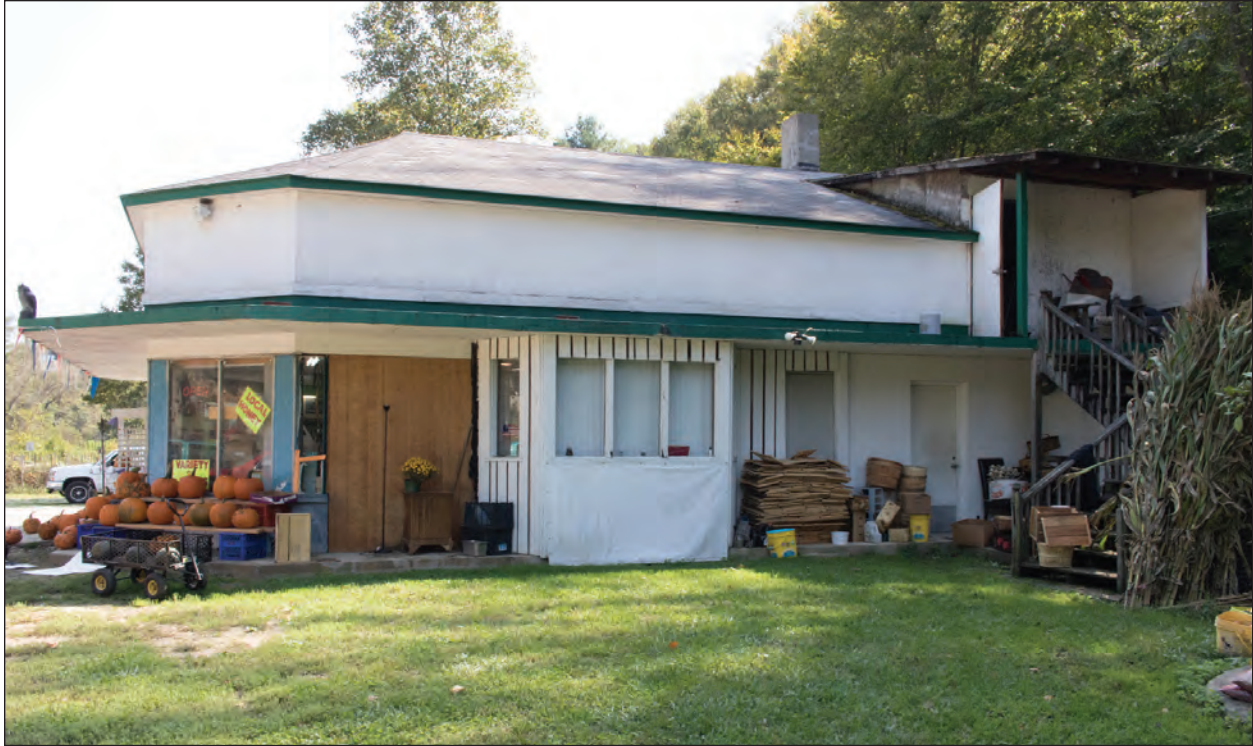
Figure 4.19. West Wall, Looking East
