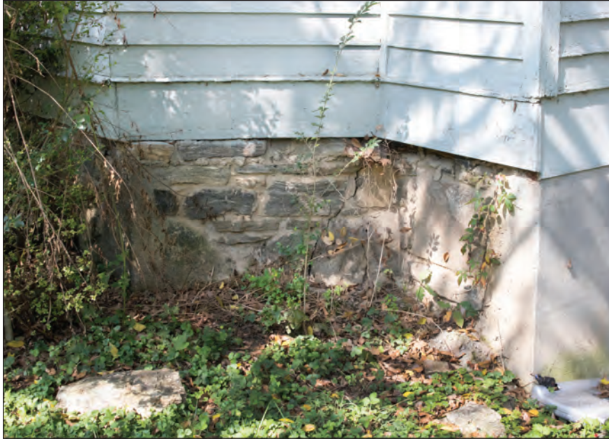
Figure 5.7. Foundation, Facing Northwest
