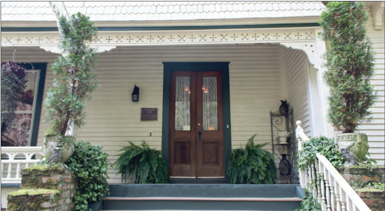
Figure 3.4. Double-Door Entrance, Facing South
