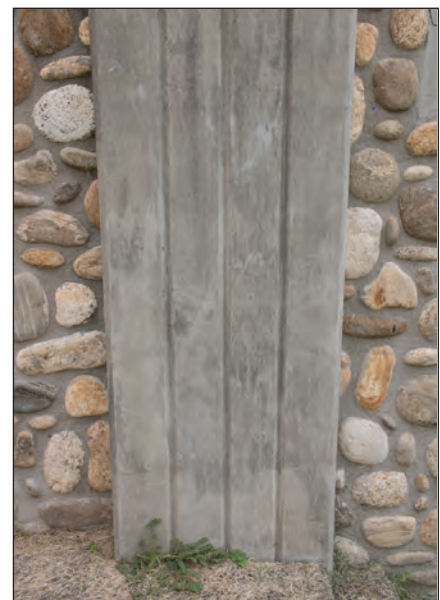
Figure 4.4. Detail of Column and Wall
