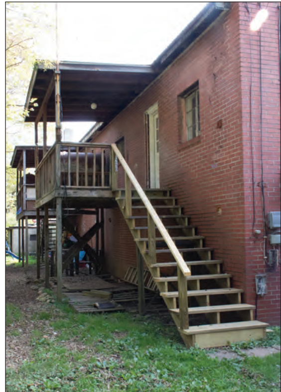
Figure 6.7. Apartment Stairs, Looking West
