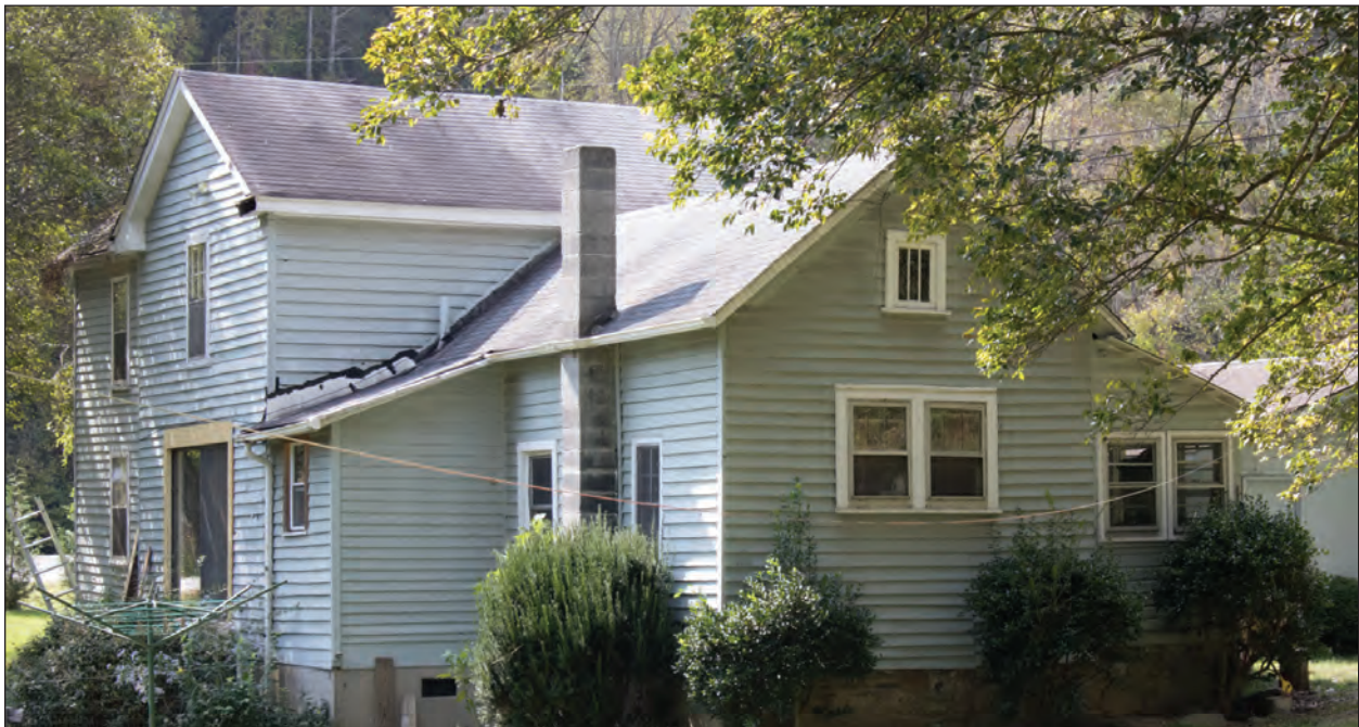
5.15. Kitchen Ell and Shed Addition, Facing Southwest
