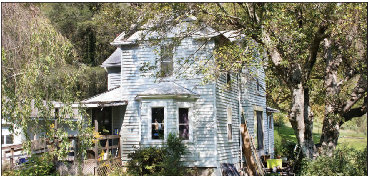
Figure 5.6. Smathers-Mease House, Facing Northwest
