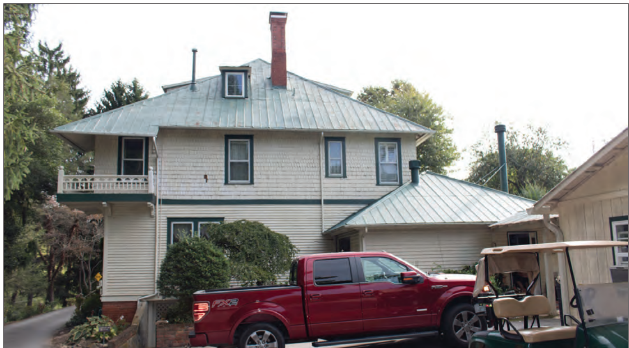
Figure 3.8. West Elevation and Kitchen Wing, Facing East
