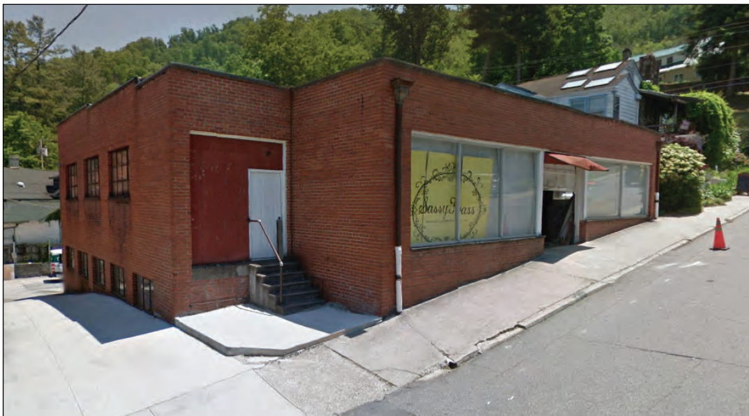
Figure 6.18. Massie Furniture Warehouse (JK0460)
