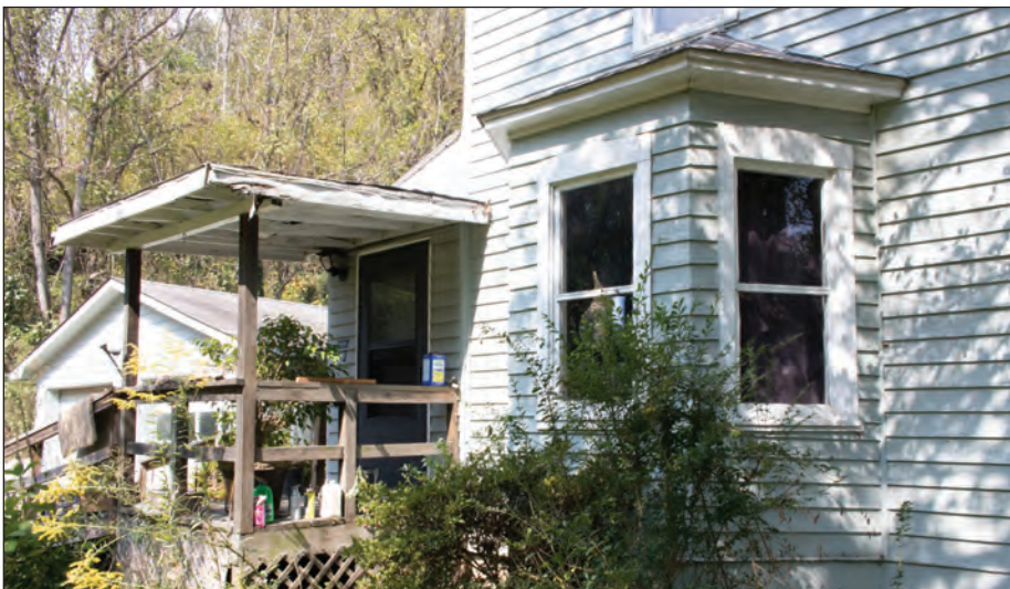
Figure 5.13. Bay Window, Facing Northwest
