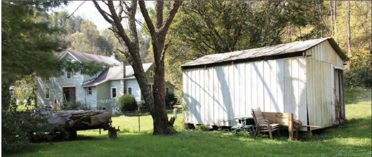
Figure 5.16. Shed, Facing Southwest
