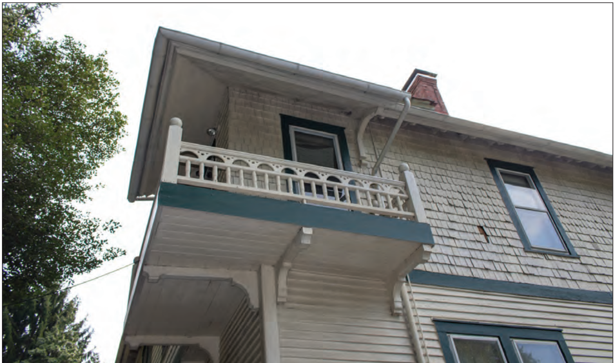
Figure 3.6. Projecting Corner Balcony, Facing East
