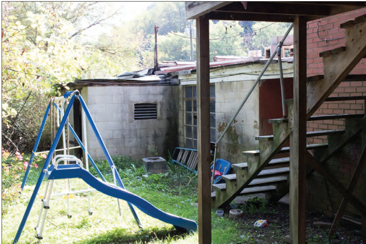
Figure 6.15. Workshop Rear Wall, Looking Southwest
