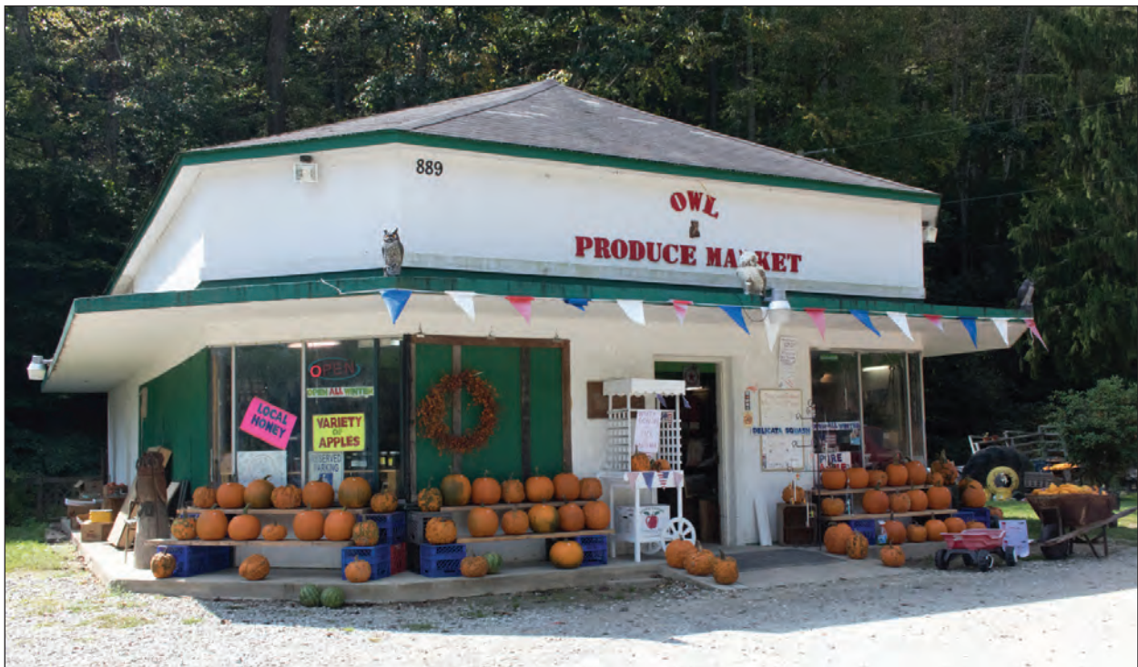
Figure 4.17. Owl Drive-In Façade, Looking Southwest
