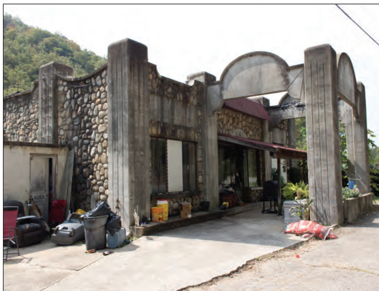
Figure 4.3. Oblique View of the Façade, Looking Southwest
