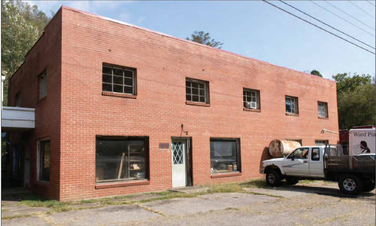
Figure 6.5. Factory Façade, Looking Southwest
