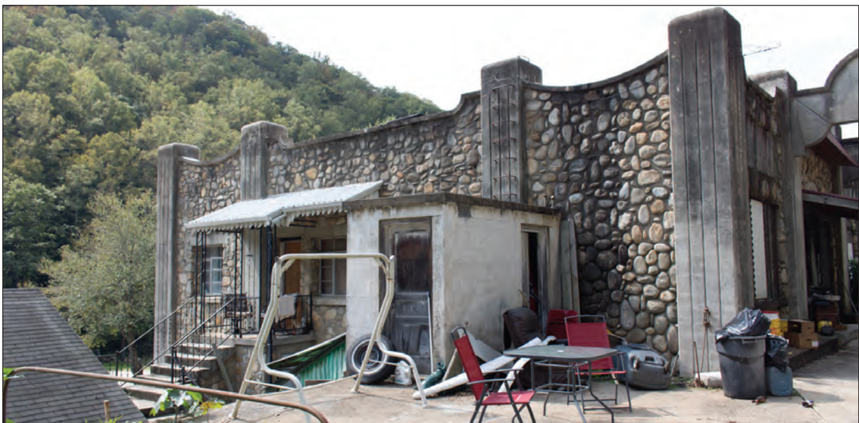
Figure 4.11. East Wall, Looking Southwest
