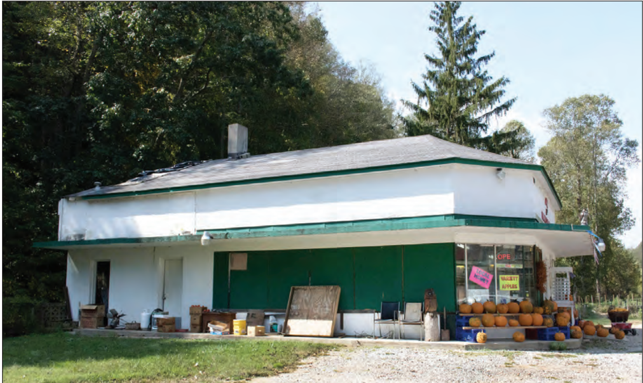
Figure 4.18. East Wall, Looking West
