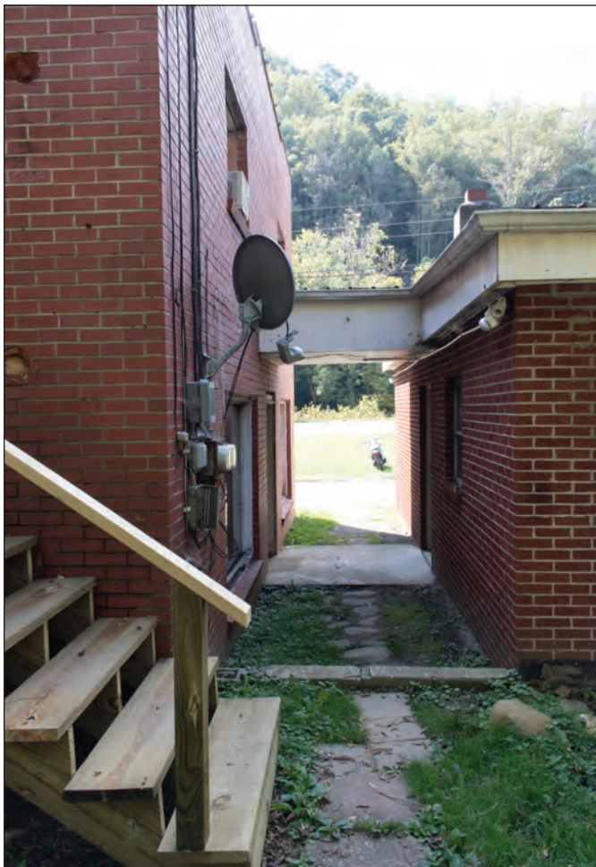
Figure 6.11. Breezeway Between Factory and Showroom, Looking North
