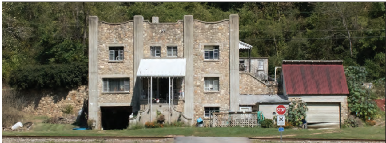
Figure 4.2. The Owl Restaurant, as Seen from South of US 19/23, Looking North
