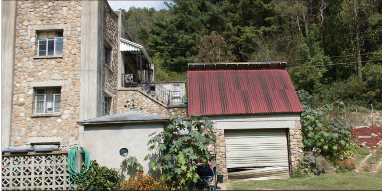
Figure 4.12. East Wall Additions, Looking North
