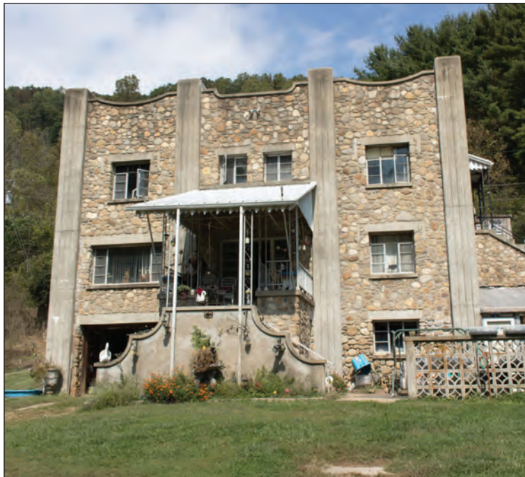
Figure 4.13. South Wall, Looking North
