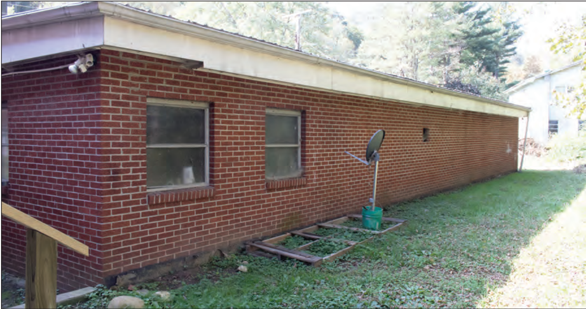
Figure 6.12. Rear Wall of Showroom, Looking East
