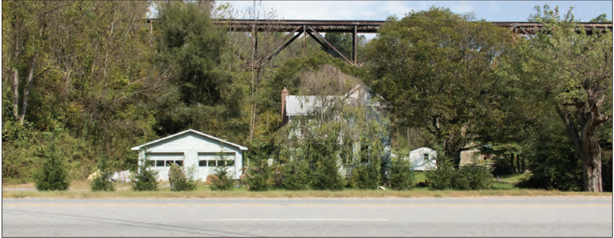
Figure 5.2. Smathers-Mease Property, Facing North
