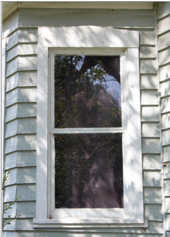
Figure 5.10. Sash Window, Facing Northwest
