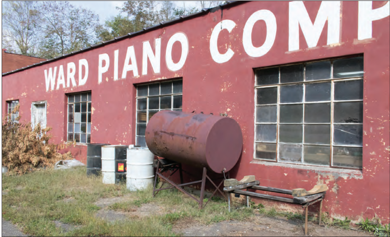
Figure 6.14. Workshop Window Detail, Looking Southeast
