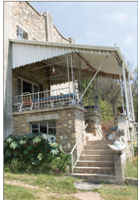
Figure 4.14. Rear Porch, Looking East
